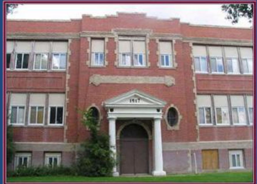
Old Burns High School, Demolished in 2005
