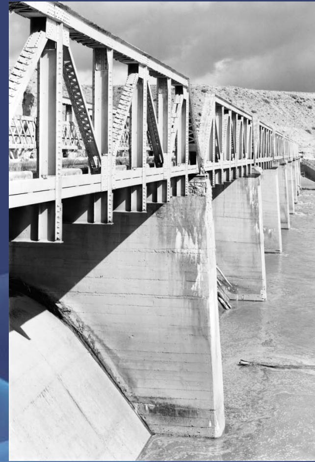
Diversion Dam in Fremont County
