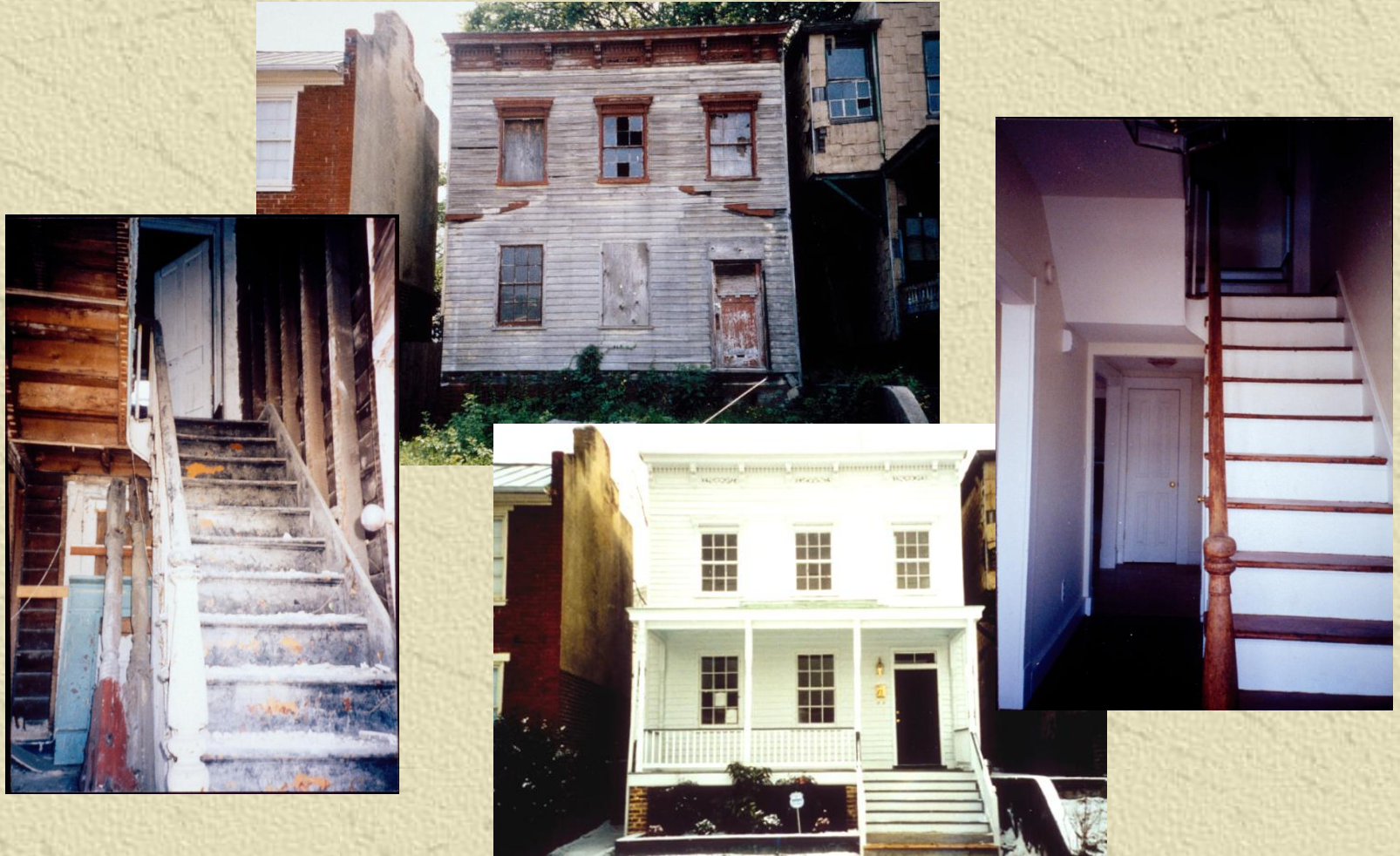
Before and After Views: House in Richmond, VA
