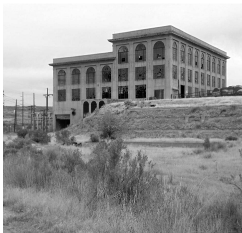
Salt Creek Oilfield Powerplant, 2010, image courtesy of Anne Toxey.
