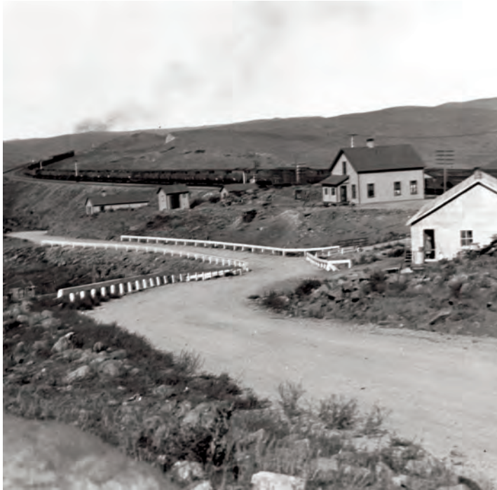
Left: Figure 31. This 1921 photograph of the Lincoln Highway through Granite Canyon shows a graded dirt road with some gravel surfacing.
