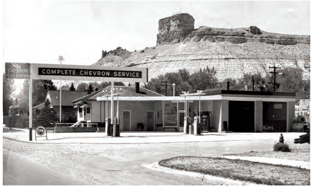
Figure 85. Oil companies modified the standard oblong box in a variety of ways, such as orienting the primary elevation at a right angle, as at this Chevron Station in Green River. Porcelain and glass façades were easily lit at night for around-the-clock sales appeal. Large display windows facilitated selling through point of purchase display. Credit: Sweetwater County Historical Museum
