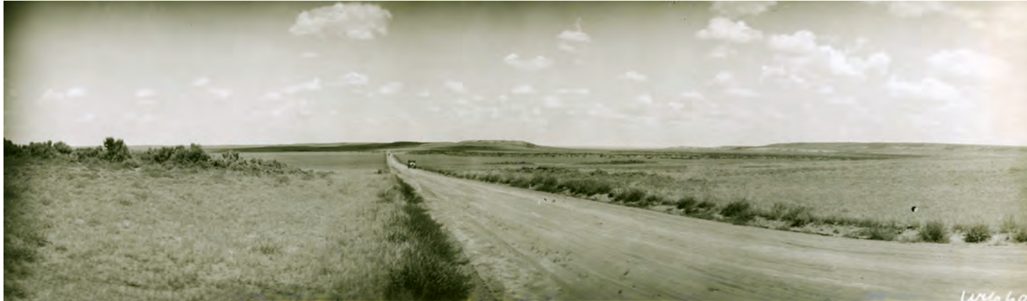
Figure 23. This 1922 photograph of the Lincoln Highway shows a section of highway west of Wamsutter that utilized an old Union Pacific railroad grade. Credit: University of Michigan Library Digital Collections, Lincoln Highway Digital Image Collection
