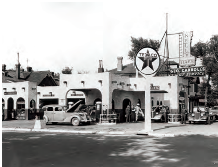
Top: Figure 82. By the late 1920s the gas station was evolving into a hybrid of filling station and repair garage—the neighborhood service station. Texaco built service stations with canopies in Wyoming and other Western states. This station in Cheyenne expressed the Mission Revival style through its use of stucco and non-structural vigas. Credit: Wyoming State Archives
